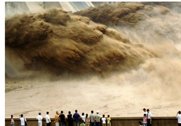
Sediment flushing of Xiaolangdi reservoir (Source: Xinhua)
